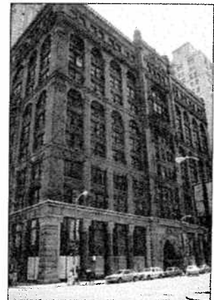
Image 18: (top) Burnham & Root's Monadnock Building touted as the tallest building in the world at the time of completion in 1891. Image 19: (bottom) Burnham & Root's Romanesque Revival style Rookery Building.
